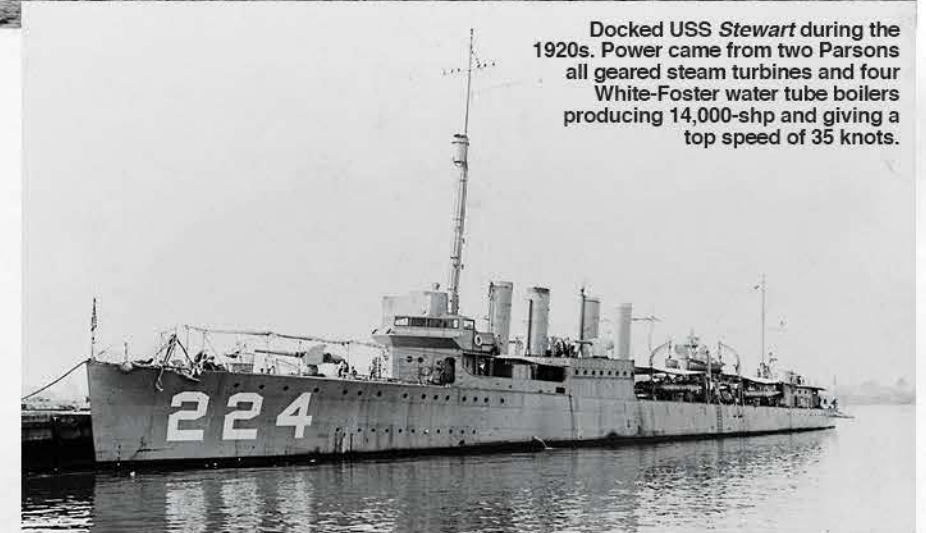
USS Stewart at high speed during the late 1920s. The Clemson -class destroyer had a length of 314-ft 5-in, beam of 31-ft 9-in, and a draft of 9-ft 4-in.
