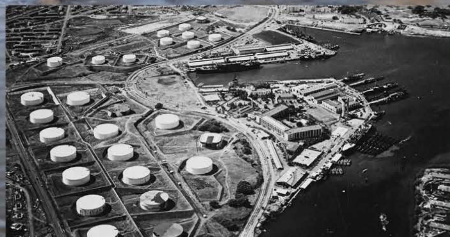
Aerial view of the Pearl Harbor Submarine Base (right center) with the Upper and Middle Tank Farm groupings at left, looking south on 13 October 1941. Among the 17 fuel tanks in the Upper Tank Farm group and 10 tanks in the Middle Tank Farm group, two have been painted to resemble buildings (topmost tank in upper group and rightmost tank in lower group).
