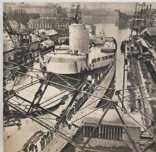
Richelieu under construction. Ready to depart France was a battle against time as advancing German troops neared Brest.
