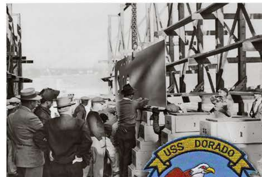
The keel of the Dorado being laid on 27 August 1942.
