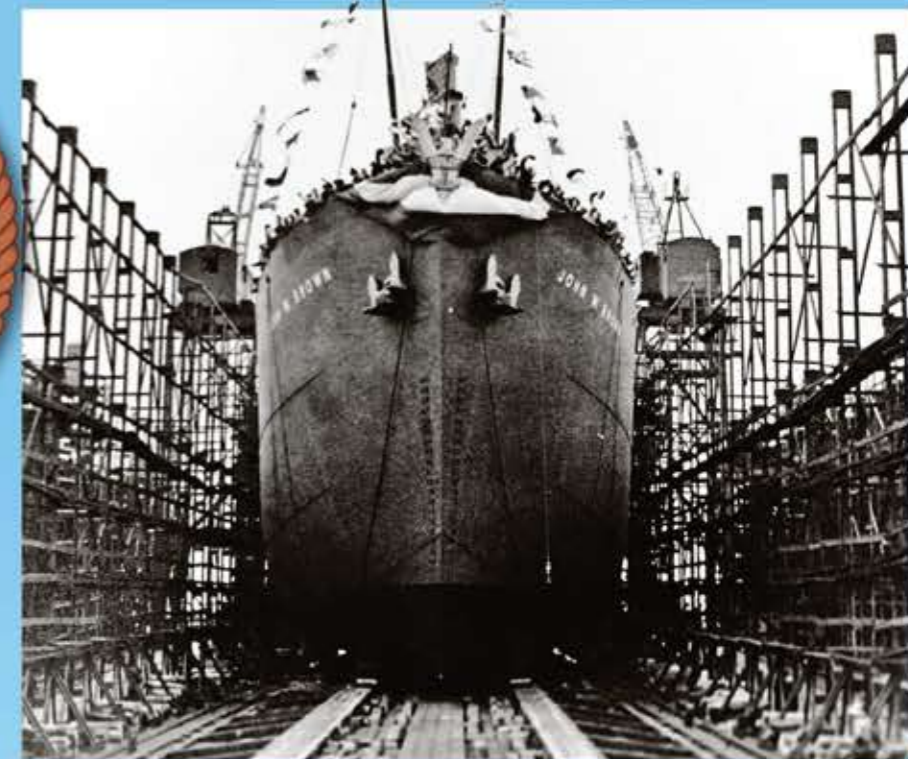
The SS John W. Brown being launched. The Liberty Ship is heading towards its 81st birthday this coming September. The vessel was ordered as an ECS-S-C1 Maritime Commission Emergency Cargo Ship, hull number 312 on 1 May 1941.
