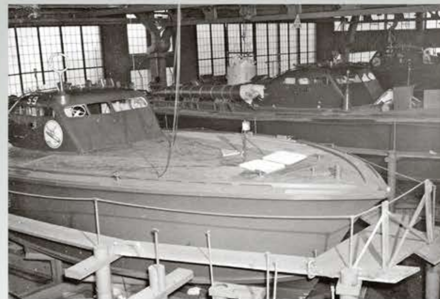
PT-59 under construction in the foreground at Bayonne, New Jersey, with PT-58 and PT-57 in the background.
