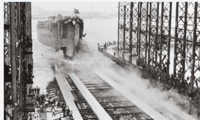
To give an idea of the pace of war-time construction, while the USS South Dakota (BB-57) is launched on 7 June 1941, at New York Shipbuilding Yard, the keel plate of USS Santa Fe is being swung into the building ways.
