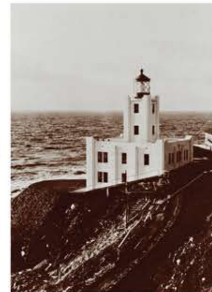
The Scotch Cap Light was an impressive concrete, steel-reinforced building but no match for the tsunami that would destroy the area.
