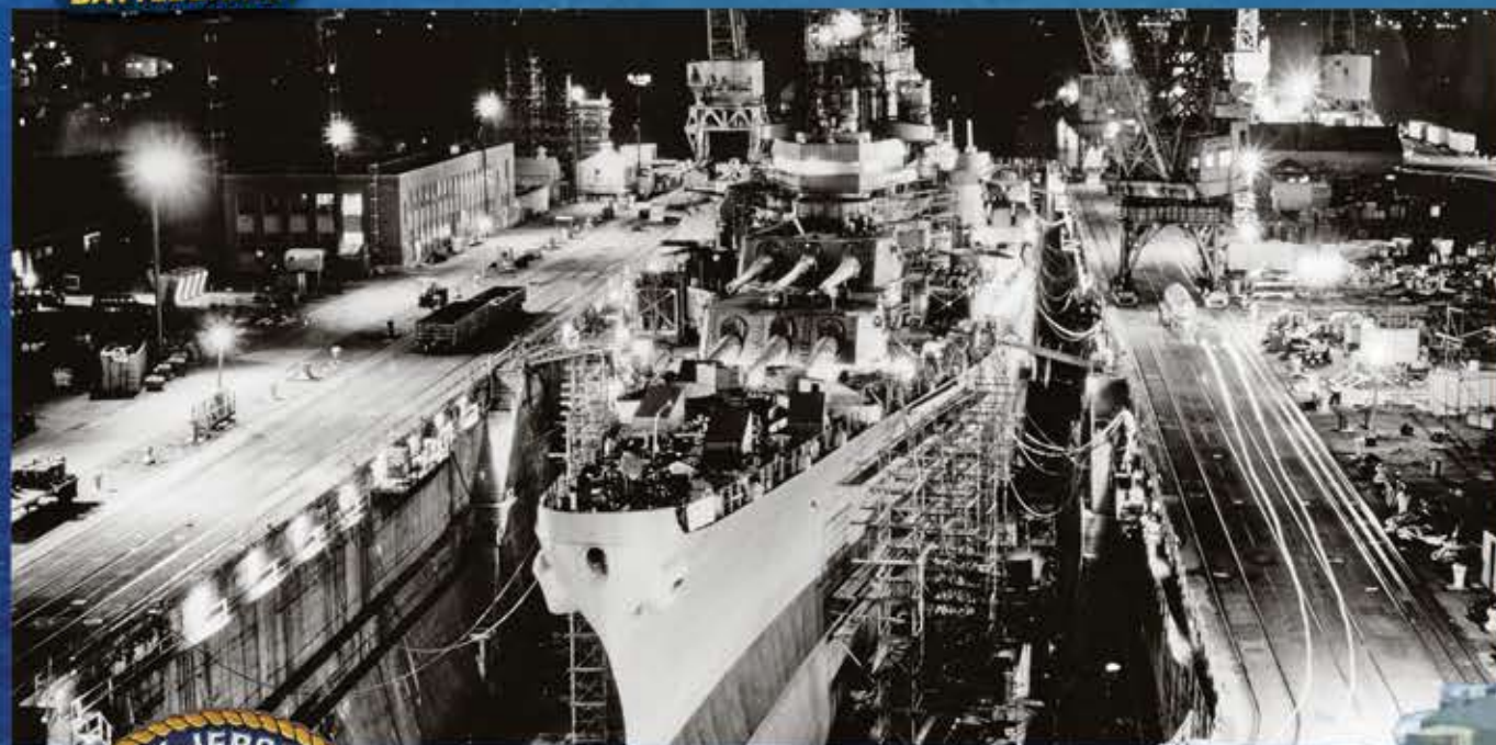
New Jersey in dry dock as modernization work is underway to prepare the battleship for a new war.
