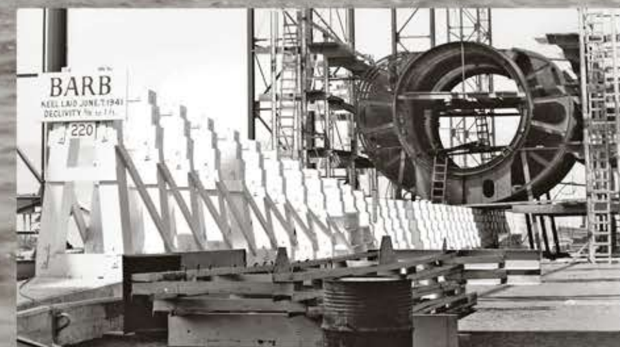
Construction begins on Barb .
