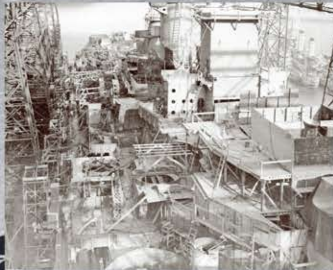
Missouri during November 1943, just two months before launch. The hull is complete up to the main deck and much of the superstructure is in frame. Amid the maze of scaffolding, air hoses, and welding leads, splinter protection for the lightweight 40mm anti-aircraft battery is being installed and the teak deck is being laid.
