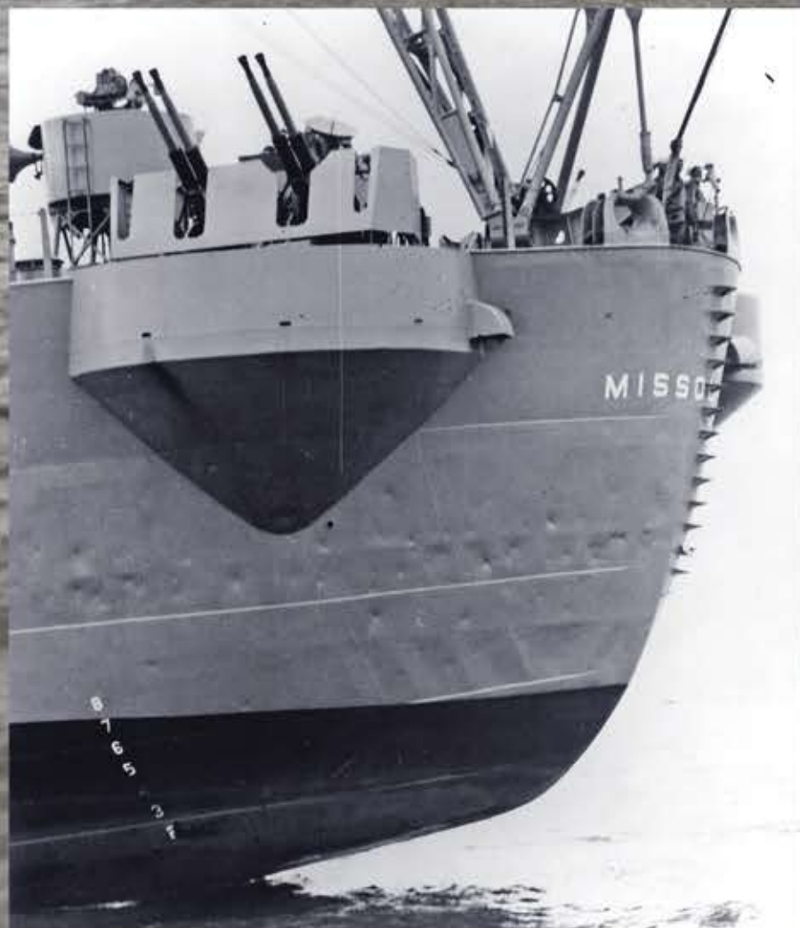
View of Missouri's stern, showing how far it was raised above her normal waterline while grounded at Thimble Shoals. This also presents an excellent view of her aft 40mm weapons. For the final freeing operation on 1 February, two windlass-type beach salvage ships — Windlass and Salvager — were linked to the Missouri by tow cables and hauled against beach gear cables that were anchored astern. Five sea-going tugs, held together by a lead tug and two harbor tugs pressing from opposite sides, worked in a surging or rocking pull.
