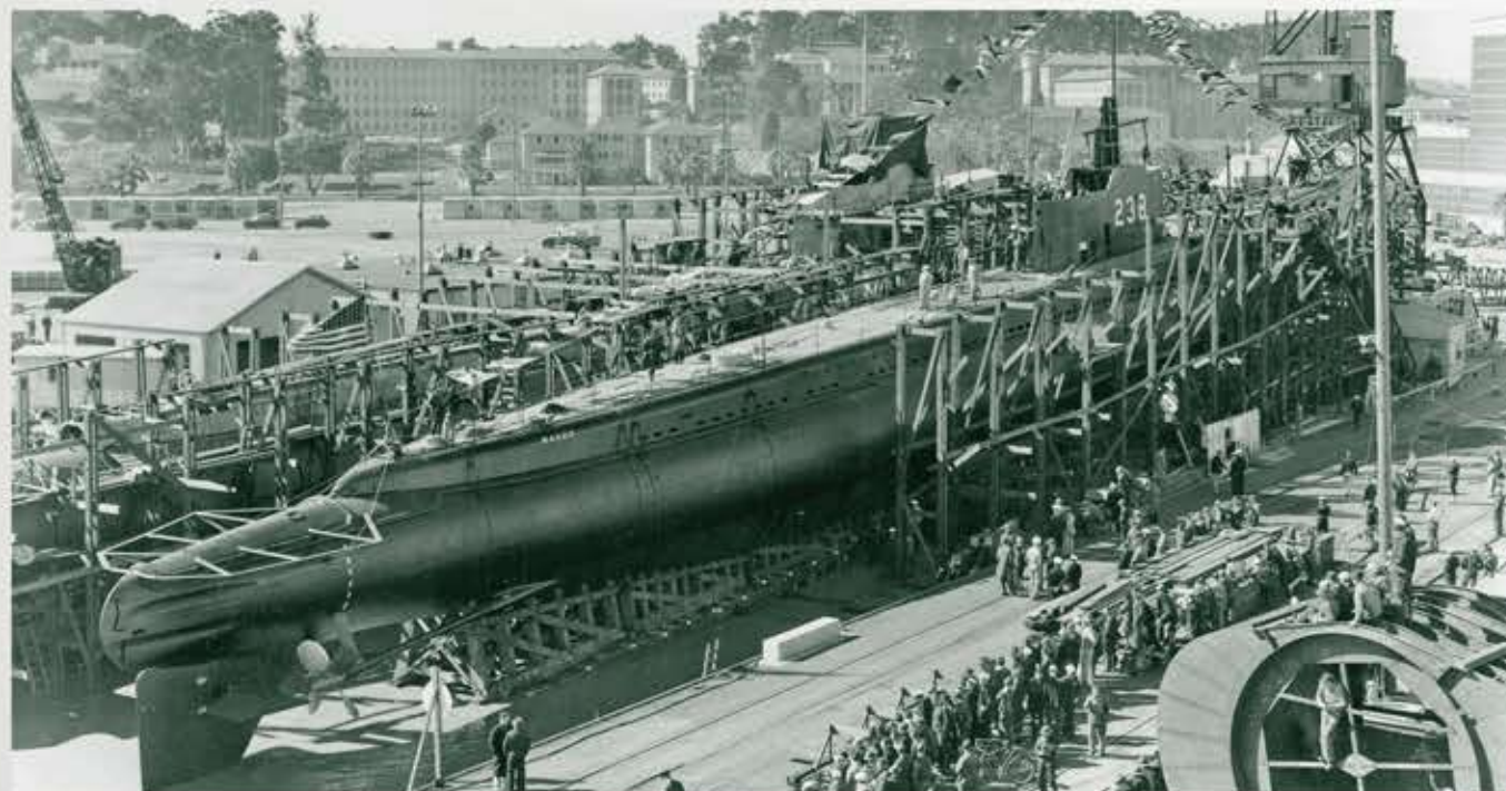
Wahoo readied for launch on 13 February 1942 at Mare Island. The Whale (SS-239) is on the building ways on the left and a hull section for Tinosa (SS-283) is just visible on the lower left corner of the photo.
