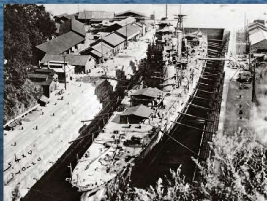
The cruiser under construction.
